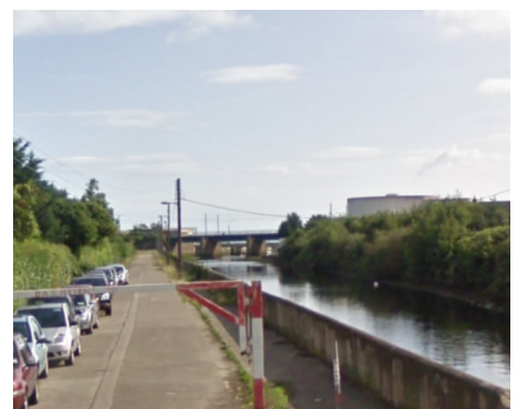
View of the existing railway bridge from Fran O'Toole Bridge
