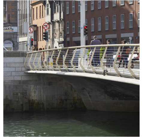
The Rosie Hackett Bridge, Dublin, by Sean Harrington Architects. Note the use of stainless steel balustrade posts.
