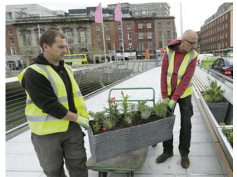
The Rosie Hackett Bridge. Note the changable inserts for the planters, for ease of maintenance.
