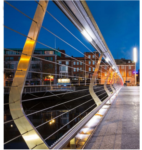
The Rosie Hackett Bridge, Dublin, by Sean Harrington Architects. Note the use of down lighting (for deck illuminance) within the handrail and uplighting (for facial recognition) at the edge of the deck.
