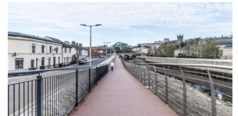
Flood defence scheme and boardwalk west of Fran O'Toole Bridge.
