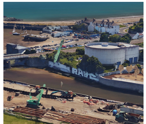
Aerial view of existing Irish Water works on south bank of the river
