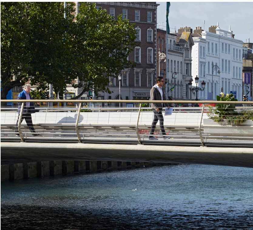
The Rosie Hackett Bridge, Dublin, by Sean Harrington Architects. Note the use of the near-transparent balustrade infill using horizontal cable.
